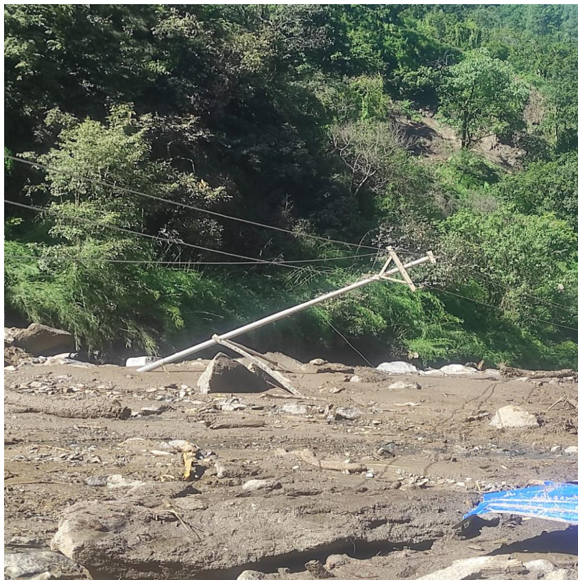
Figure: Damage of Transmission Line Network
