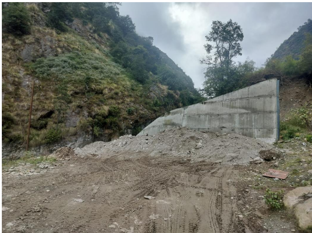
Figure: Backfilling work at Headworks site
