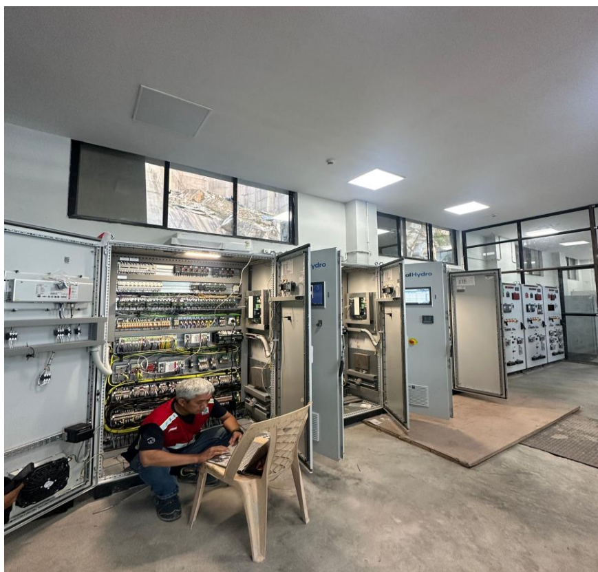
Figure: Switch Gear Panel
