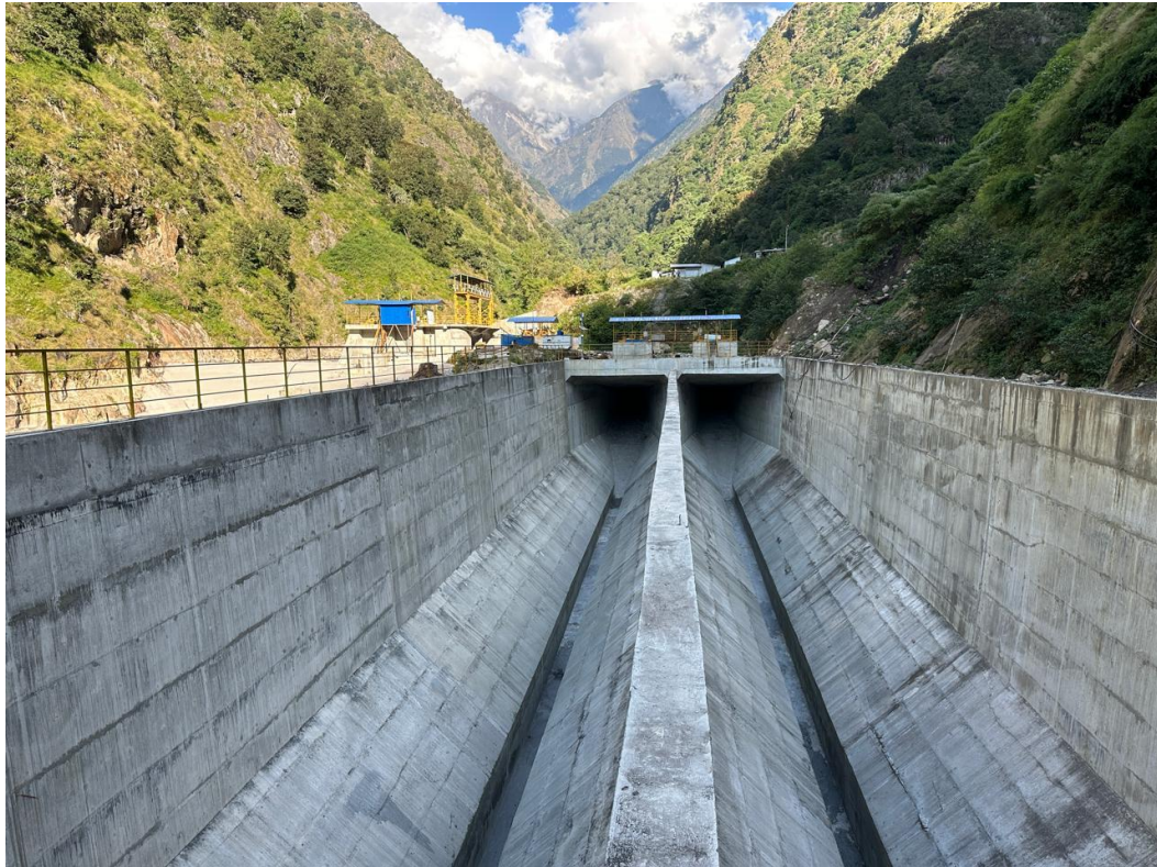
Figure: Settling Basin
