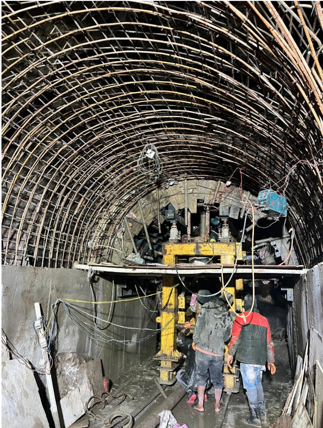
Figure: Adit Right Wing Concreting
