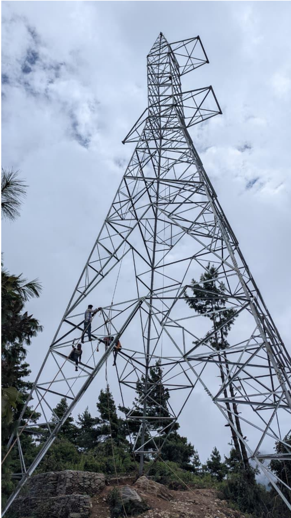
Figure: Completion of AP10 erection
