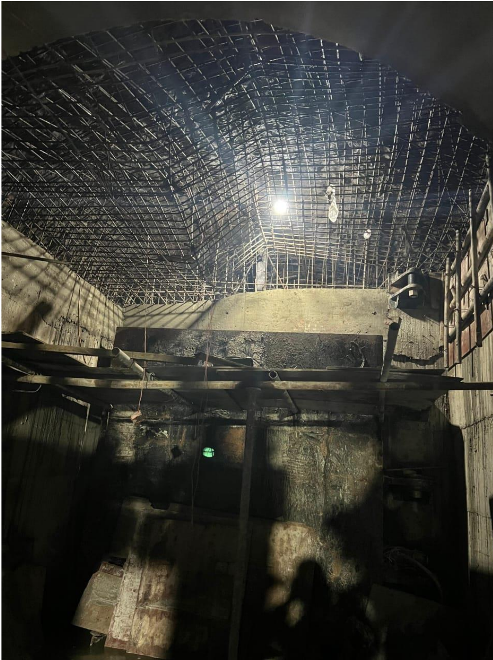
Figure: Bulk Head
