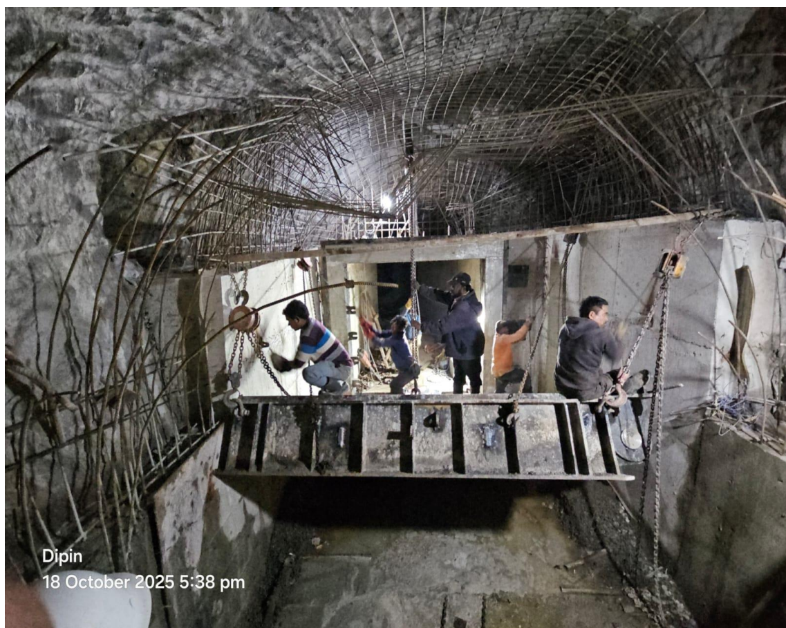
Figure – Bulkhead gate Erection completed.
